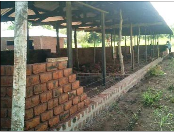
Each row of bricks is carefully put in place
